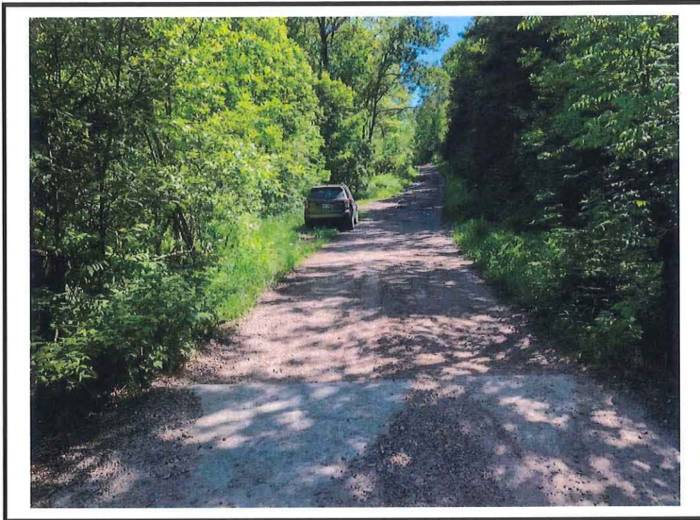
Photo 3 East approach from centre of structure
