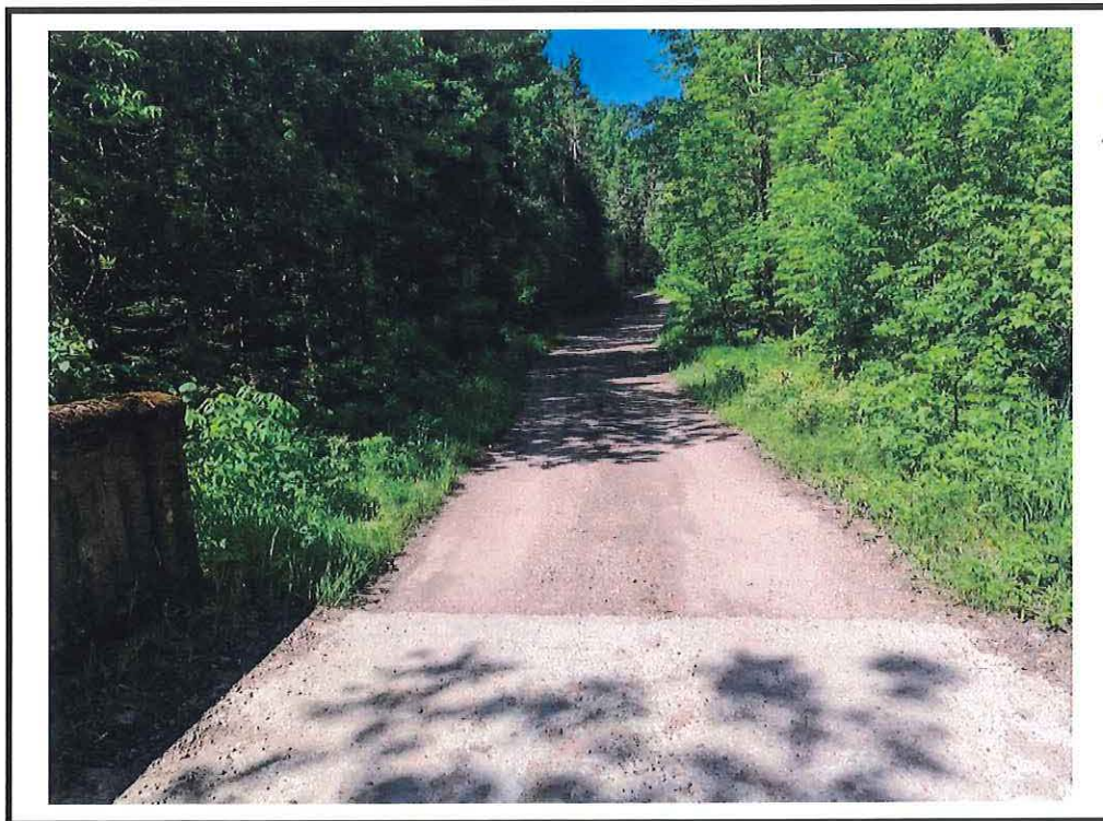
Photo 4 West approach from centre of structure
