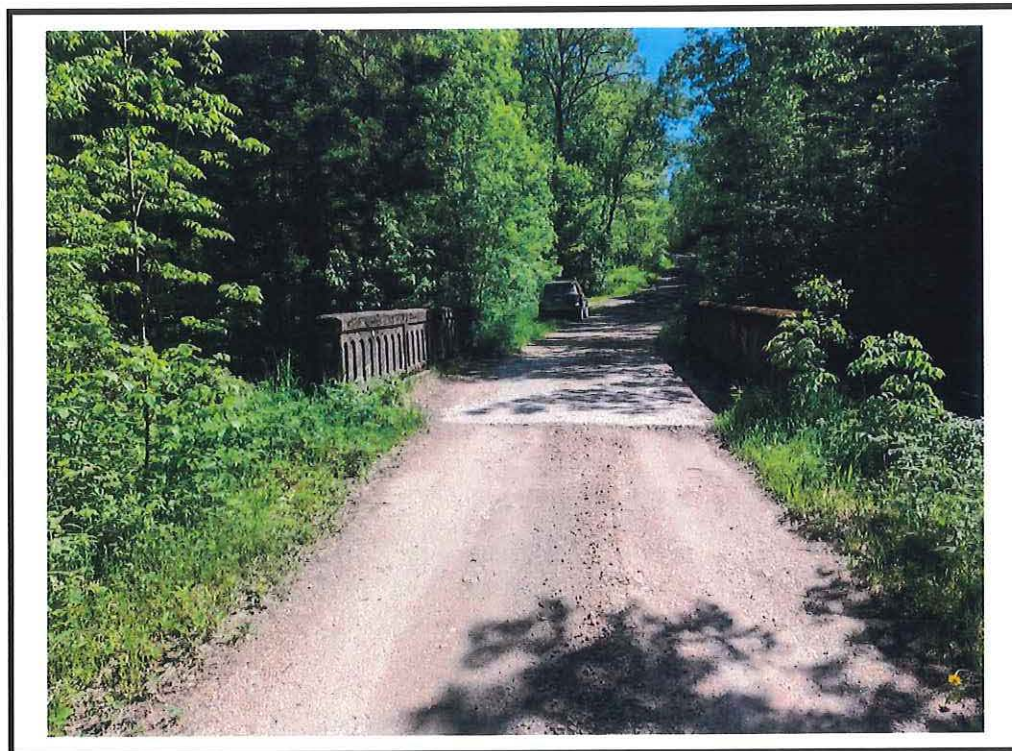
Photo 2 Structure from west approach
