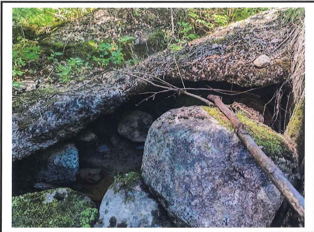
Photo 18 Concrete slope protection at southwest corner failed
